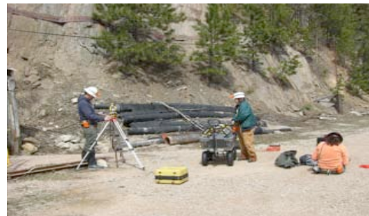
Figure 1: Preparing for the Laser Survey of the 300L in April
